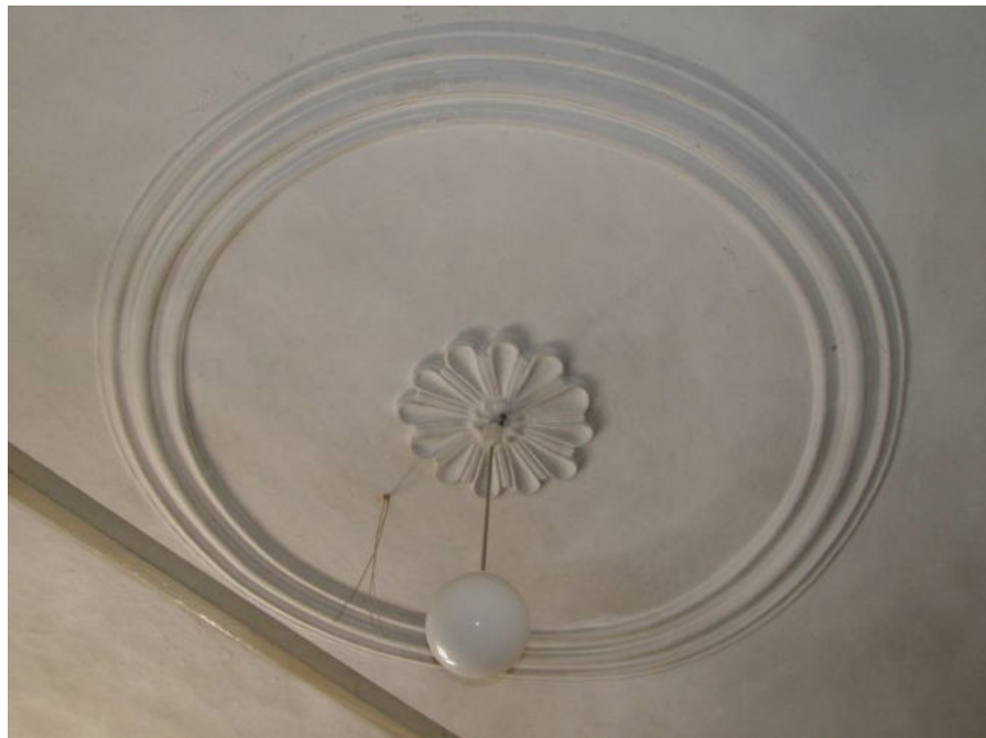
36. Detail stropu 2.NP
